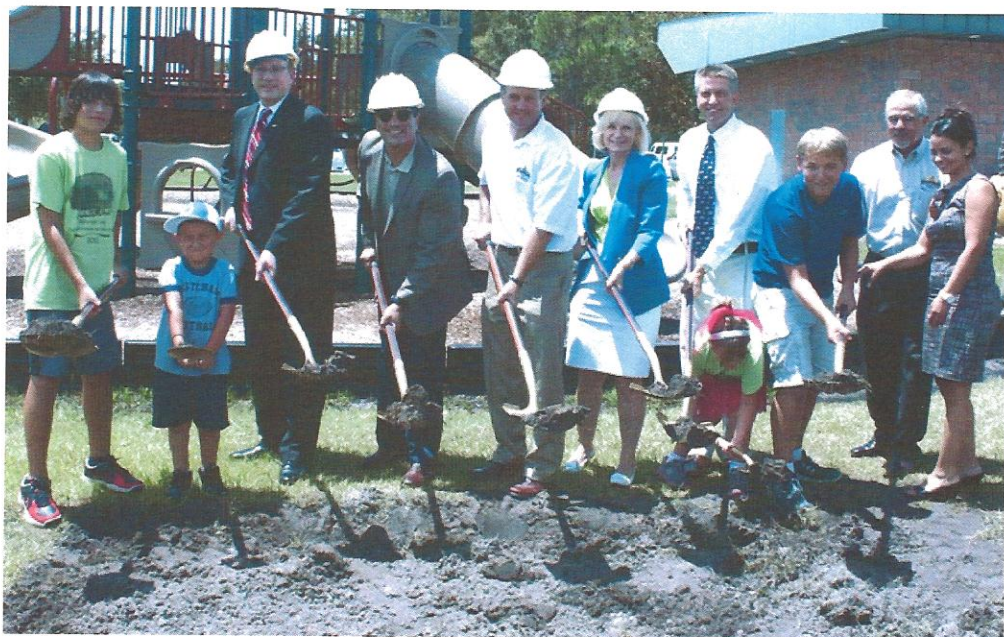
Commissioner Sandy Murman helped break ground for the Westchase Park multi-purpose Gymnasium at a special ceremony held at the park's recreation center. Westchase children, parents, volunteers and park staff were on hand as they celebrated the building of the gym. Click on the following link to see a video of the event: http://youtu.be/wW0-qWjTRdI
